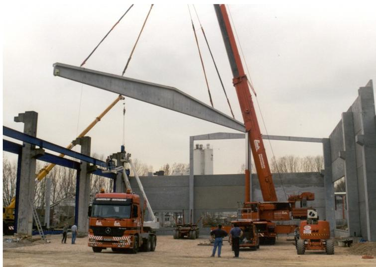
Figure 1.3: Assemblage of a 40 m roof girder
