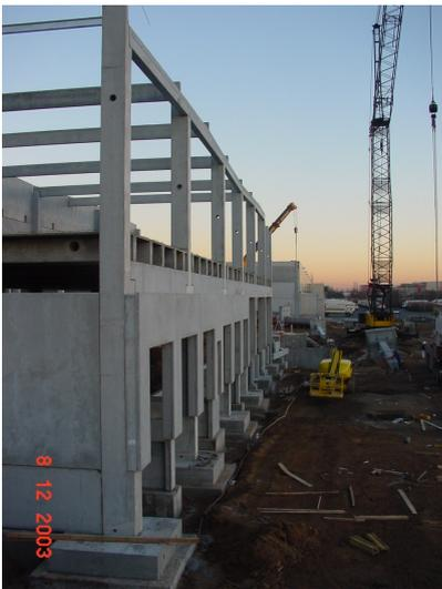
Figure 1.1: Industrial precast concrete building
