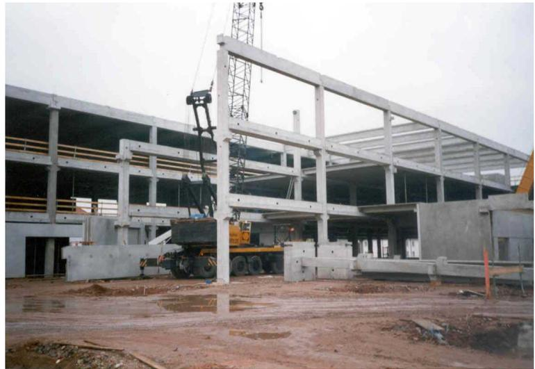
Figure 1.2: Industrial precast concrete building (distribution centre)
